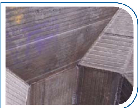
Vidaplate V45 chute in cement plant
